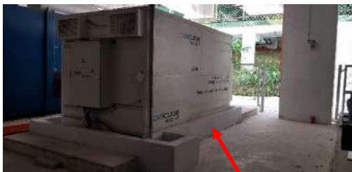
Tertiary Containment on site for Spillage Control
